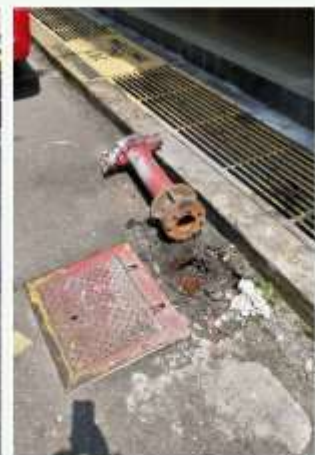
Gambar rajah 4: Pili Bomba Patah
