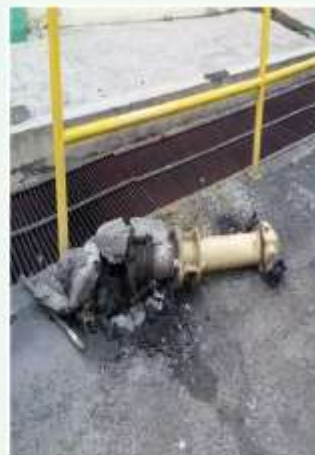
Gambar rajah 4: Pili Bomba Patah
