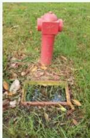
Gambar rajah 3: Pili Bomba Bocor
