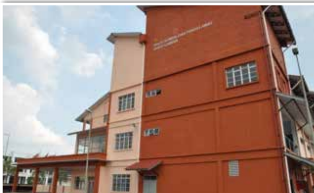
BBP BUKIT GAMBIR, JOHOR Fire and Rescue Station Bukit Gambir, Johor
