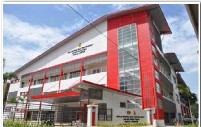
BBP JALAN HANG TUAH, KUALA LUMPUR Fire and Rescue Station Jalan Hang Tuah, Kuala Lumpur
