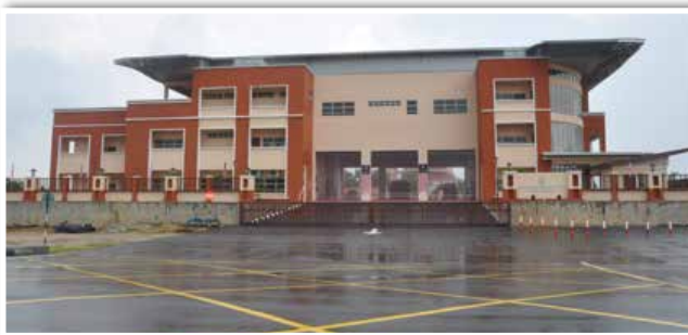
BBP JASIN BESTARI, MELAKA Fire and Rescue Station Jasin Bestari, Melaka
