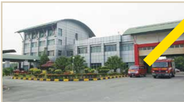
BBP KLIA/ KLIA Fire Station
